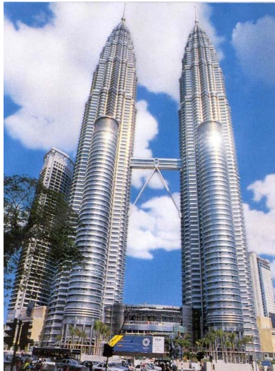
Petronas Twins Towers, Kuala Lumpur, Malaysia. 387 m.
